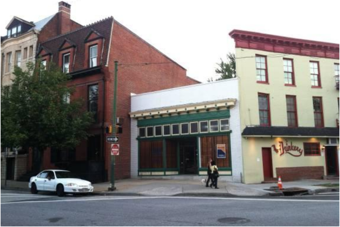
A view of the current structure
